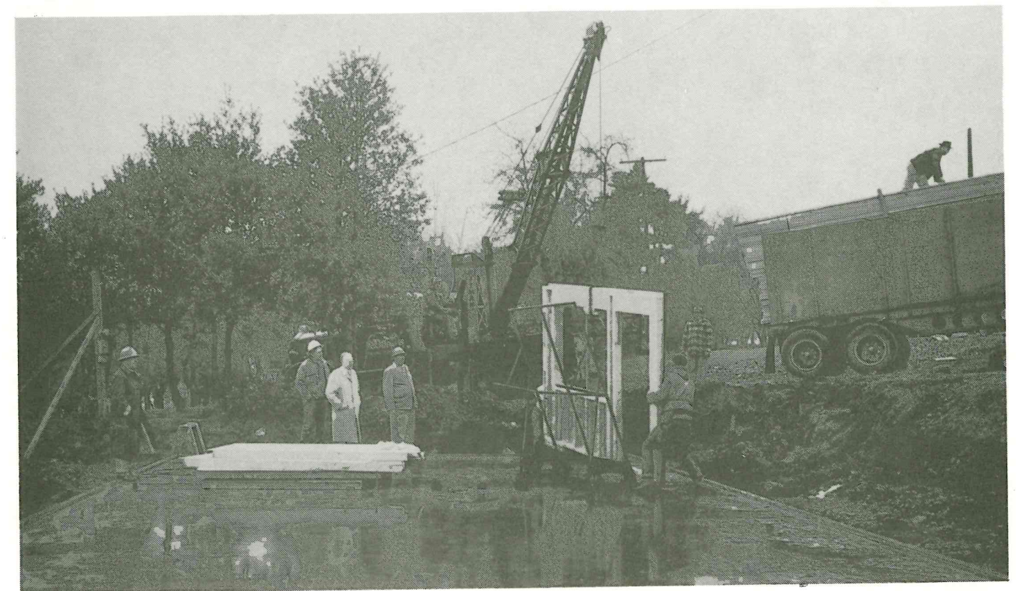
Erecting prefab sections, 1959.
